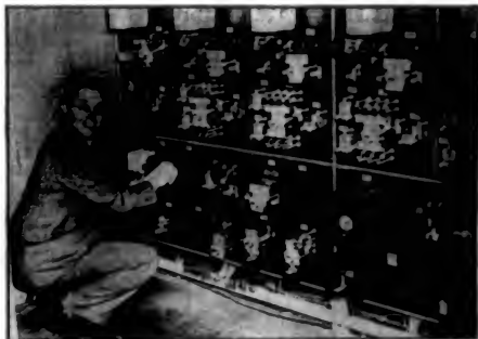
JOE WHITENHOUSE, Chief Transmitter Engineer, makes an adjustment on the largest relay panel ever employed by any commercial radio station in the United States. This relay panel, created in the WLW Research Laboratory, operates all automatic devices throughout the transmitter.
