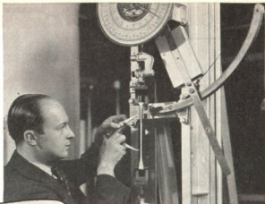
② All materials must pass severe tests. Here an engineer tests a sample of that important little item — rubber tape.
