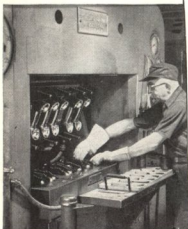
③ Moulding handles for telephone handsets—one of 248 parts in your Bell telephone.
