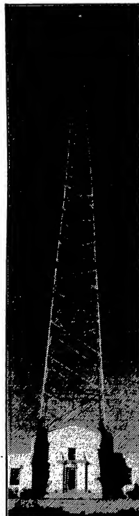
TOWERING 465 feet skyward, the KNX single mast vertical radiator is as high as the Los Angeles City Hall and is responsible for the powerful signal enjoyed by KNX throughout Western America, Canada and Alaska.
